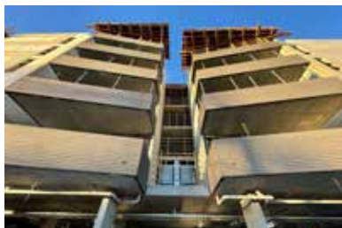
Unison's 74-apartment building in Werribee nearing completion
